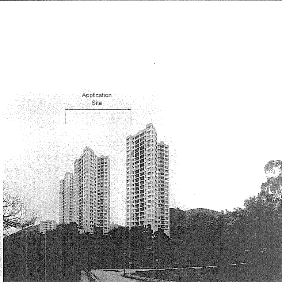
VP15: View West towards Application Site from Middle Lane with Proposed Development
