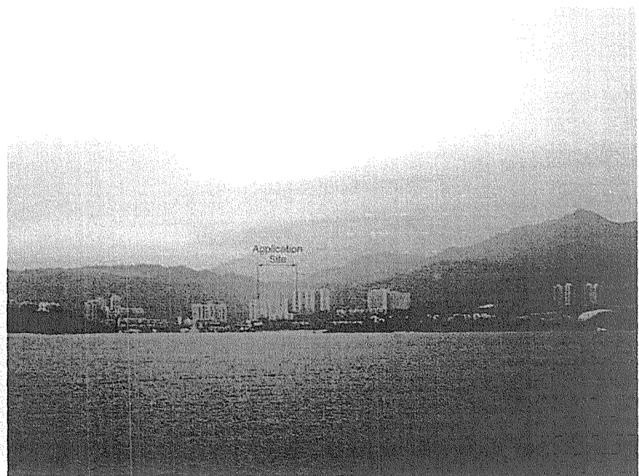
VP11: View South-West towards Application Site from the Disneyland Promenade with Proposed Development
